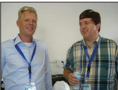
Bastiaan Lammers, left, of Boskalis Dolman with Neil Geerers of Tetra Tech at the project site.
